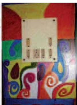
Beautifying a dirty switchboard
