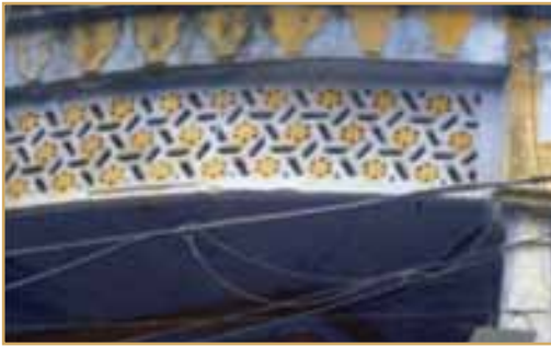
A house in Chandni Chowk
