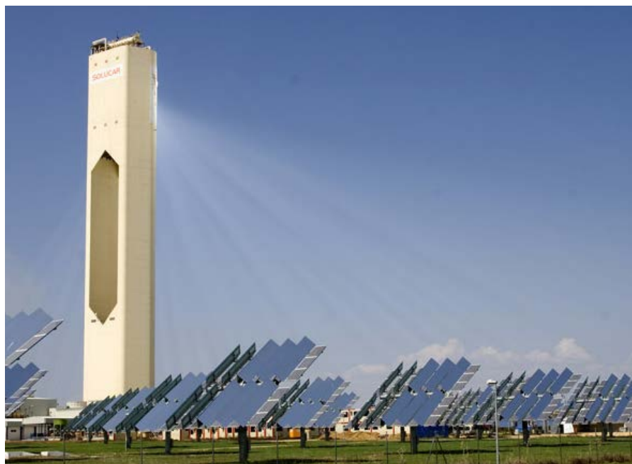
Fig. 9. A power plant in Spain uses energy from the Sun, instead of coal, to produce the steam that runs its generators. Because of the dust in the air, one can actually see the path of the Sun's rays.
